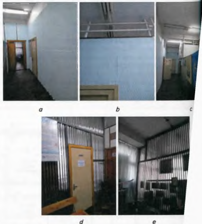
Fig. 2. Photographs of the rooms in the office of open space with partitions: 100 % separation (ceramic panels and expanded glass pipes) (a); 75 % separation (ceramic panels and expanded glass pipes) (b); 50 % separation (glass pipes with rubber gaskets) (c); 100 % separation (glass pipes with rubber gaskets) (d); 100 % separation (glass pipes with rubber gaskets) (e).
