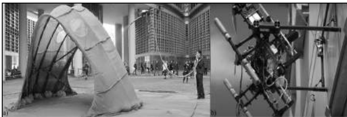
Figure 2 – Drones in construction a) – cement mixture spraying; b) – hole drilling [4]
