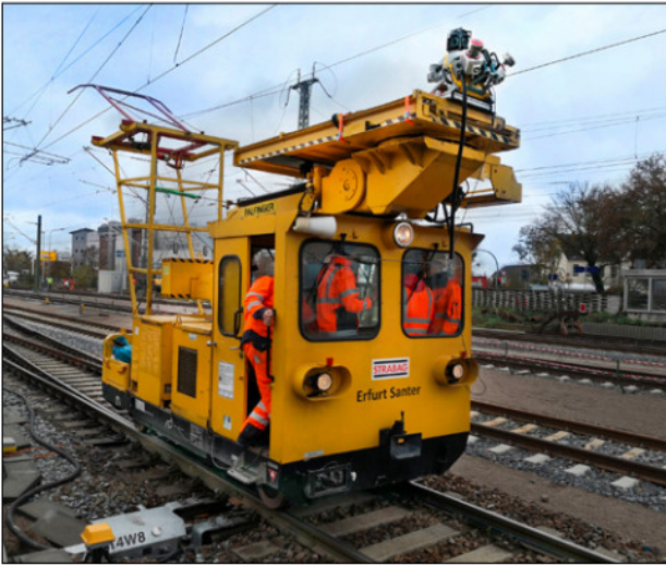
Fig.2. Installation of a mobile cartographic system on a railcar
