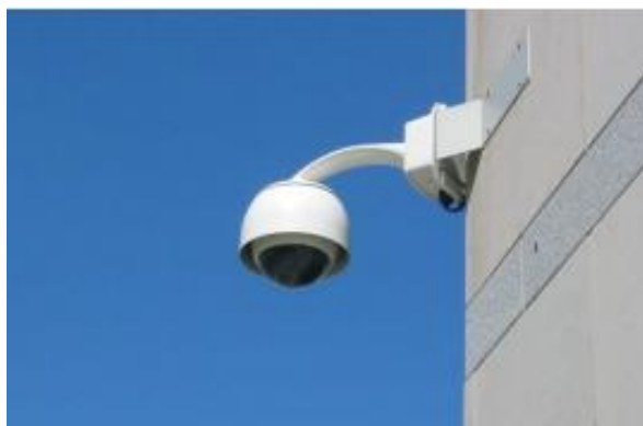
Figure 2.2 – Semi-covert CCTV camera that may have a crime prevention advantage over an overt system because offenders can never be sure in which direction that camera is facing
