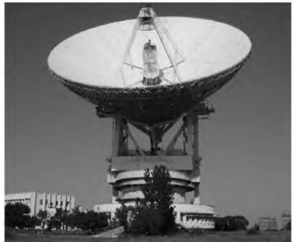
Figure 2. Yevpatoria RT-70 Antenna
